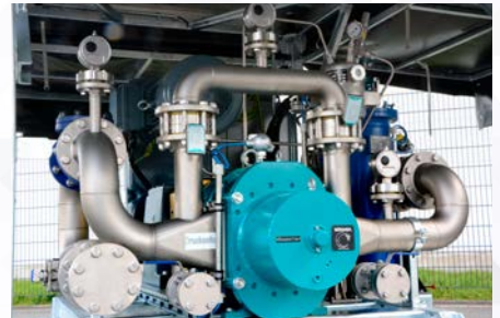
Variocap as mechanical overpressure protection
