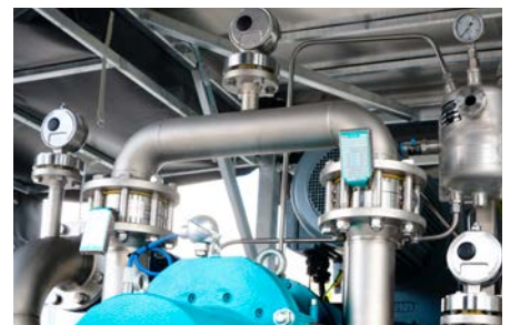
Overpressure protection by bypass with rupture disks
