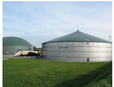
Gas-proof stretch ceiling cover (one or two layers)
