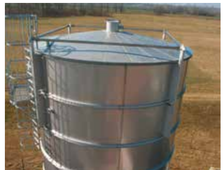
Stainless steel roof
