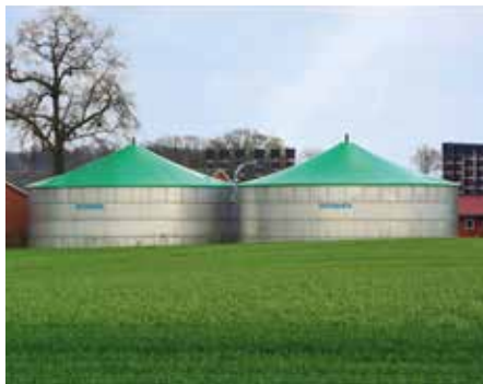
Stretch ceiling cover (one layer)
