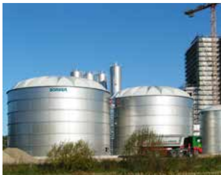
GRP roof (cupola roof)
