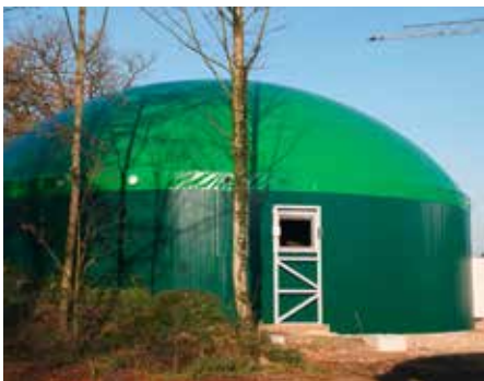
Double membrane air-supported roof
