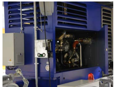
Motor with sound enclosure
