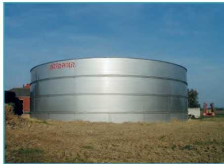
The horizontal segmental design proved to be suitable for series production and has been used to this day.
