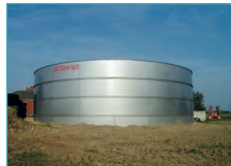
The horizontal segmental design proved to be suitable for series production and has been used to this day.
