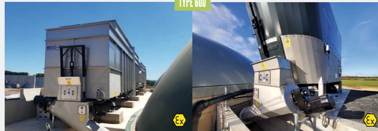
Fermenter screws TYPE 600 according to ATEX feed the fermenter directly. Both units are equipped with a slide opening for this purpose.
