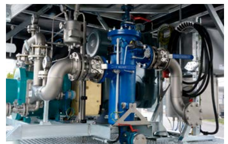
Filter system with differential pressure measurement
