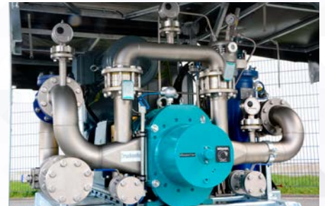
Variocap as mechanical overpressure protection
