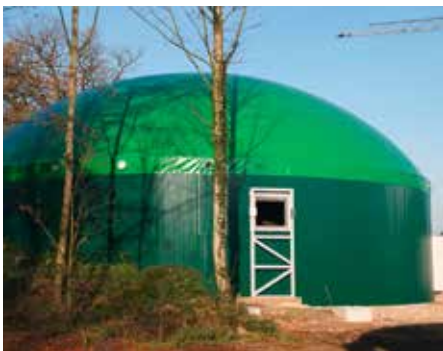
Double membrane air-supported roof
