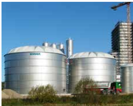
GRP roof (cupola roof)
