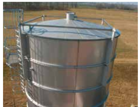
Stainless steel roof
