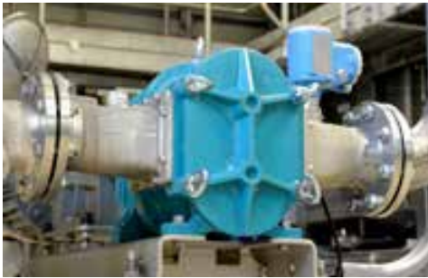
BLUEline pump for conveying cleaning agent
