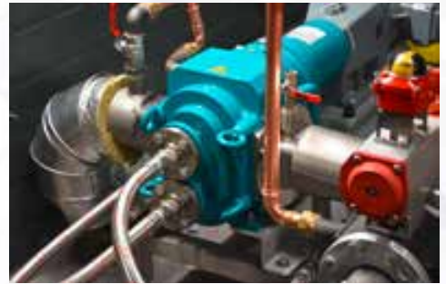
BLUEline pump with heater jacket and heater cover
